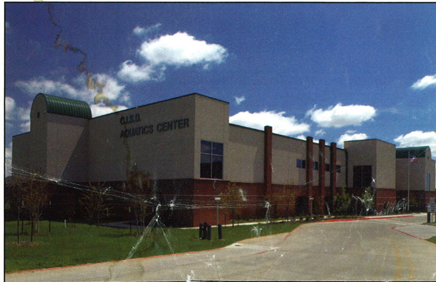
Located northwest of Dallas, in Southlake, TX, Carroll ISD's Aquatic Center features a 180-by-75-ft pool and a 30-by-40-ft warm-up pool.
